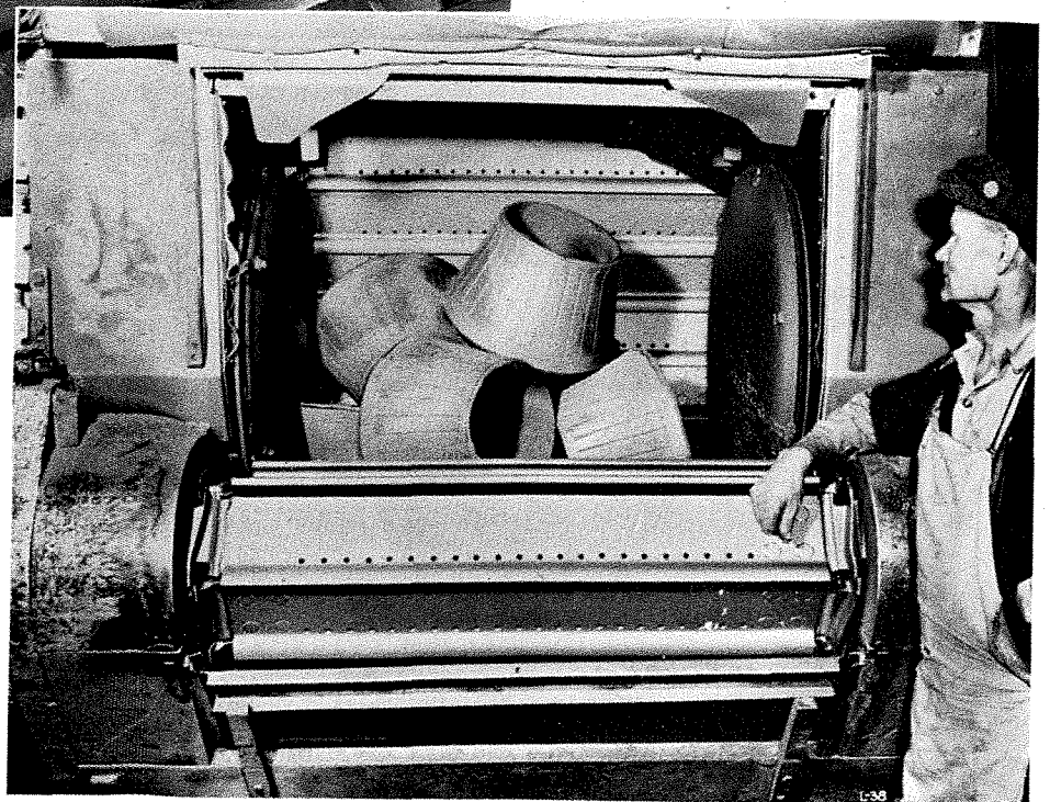
At right: General Steel Wares, London, Ontario, clean furnace upper domes in their 36" x 42" Wheelabrator Tumblast. This machine will clean large numbers of small parts, or small quantities of large parts with equal efficiency.
